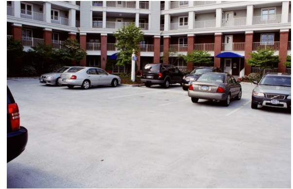
Typical upper level parking deck with waterproof, traffic bearing membrane applied to protect lower parking levels.
